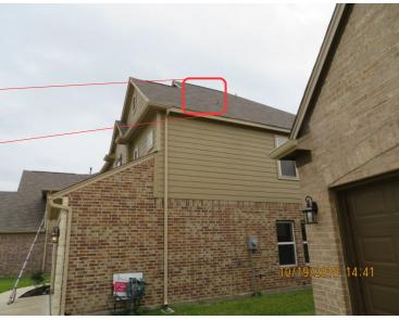
Also spotted lifting flashing and short trim on right corner. Properly repair to prevent water intrusion
