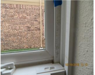
• Properly replace deteriorated caulking/mortar on exterior windows to avoid water infiltration
