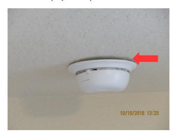
• Note: Noted only one Carbon Monoxide alarm upstairs. One alarm may not be sufficient for both sides/hallways. Code states: Carbon Monoxide alarm required immediately outside each sleep room. Install for personal safety
