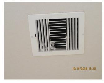
• Maintenance Tip: Routinely, clean inside intakes, ducts, and routinely replace filters to protect evaporator coil from clogging or damage.
