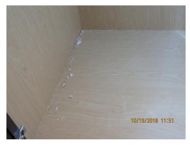
• Replace deteriorating caulking, apply caulking where missing, repair poor finish countertop surfaces.
