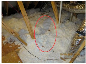
• Observed insulation in contact with an exhaust. There should be a min clearance of 1" for double wall/type "B" and 3" for single wall exhausts. In need of repair
