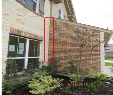
• Mortar separation in the masonry noticed in the garage area. Properly repair
