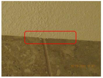
• Properly seal cracked grouts on soap holder
