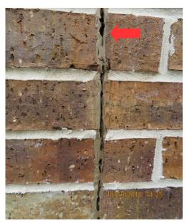
• Apply missing caulking on front exterior walls to avoid water intrusion
