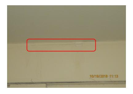
• Observed gray spots at several upstairs wall locations: bedrooms, utility room, hallway, etc. Inspector was not able to determine the source, or root cause. Consult a professional to conduct a thorough assessment, and perhaps an air quality test, moist level test, etc. Properly repair as needed
