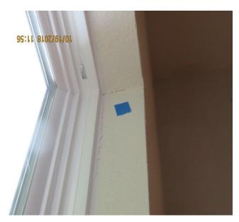
• Remove construction debris from window railing for proper drainage
